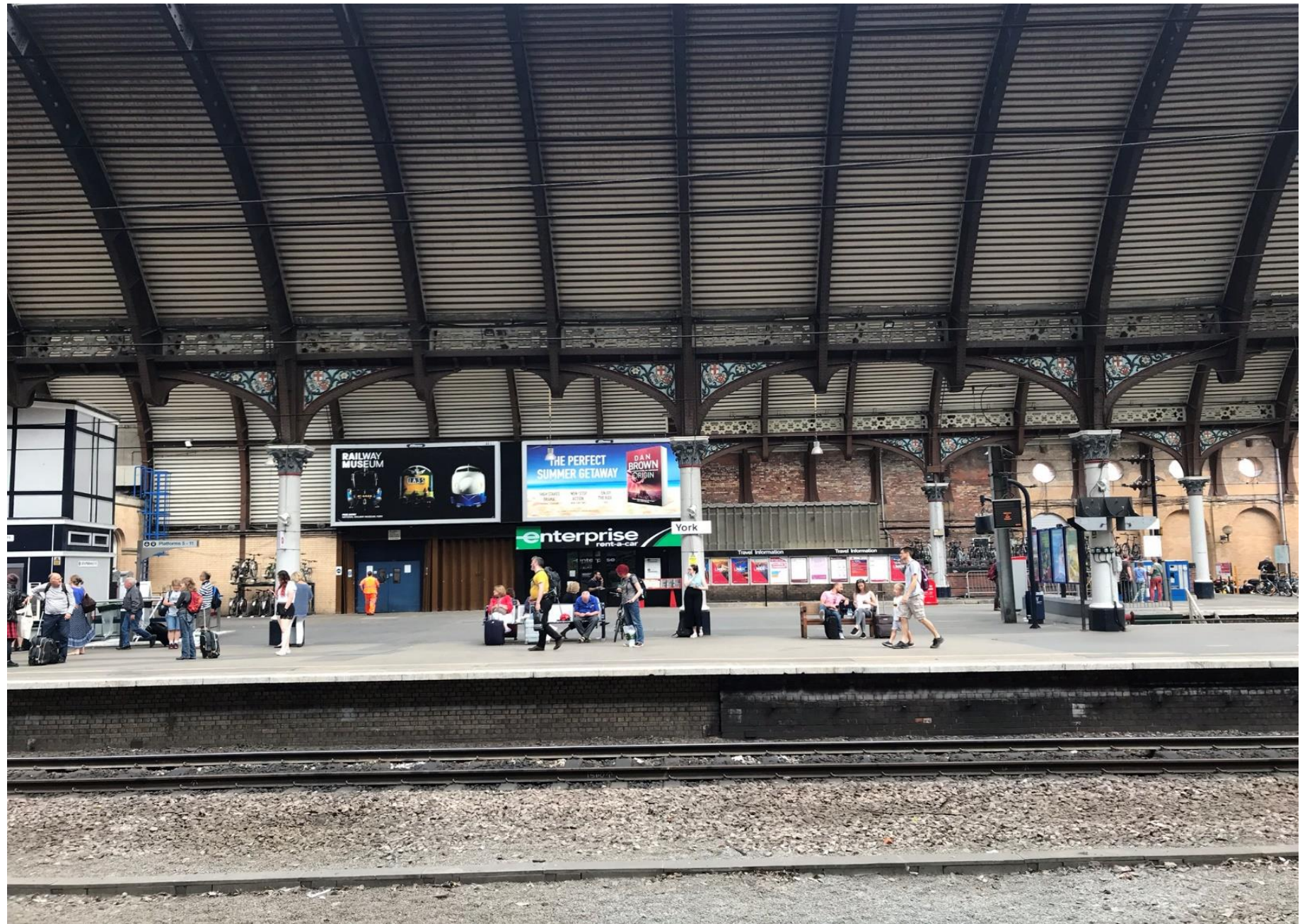
View of South Shed area
